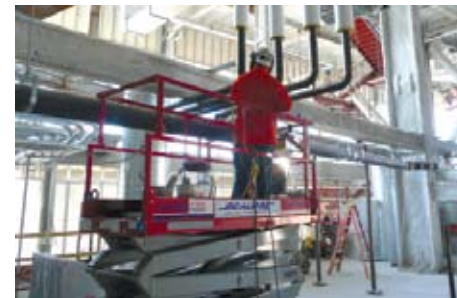
A technician works on a commercial project.
